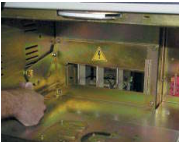
serranda cubicolo cubicle shutter
